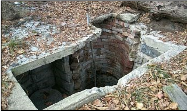
Pictured above is one of two underground brick vaults built to ferment beer.
